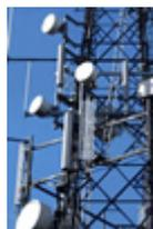
Tele communication can rely on radio waves to send messages across a nation. Here a repeater tower boosts the radio signal.
